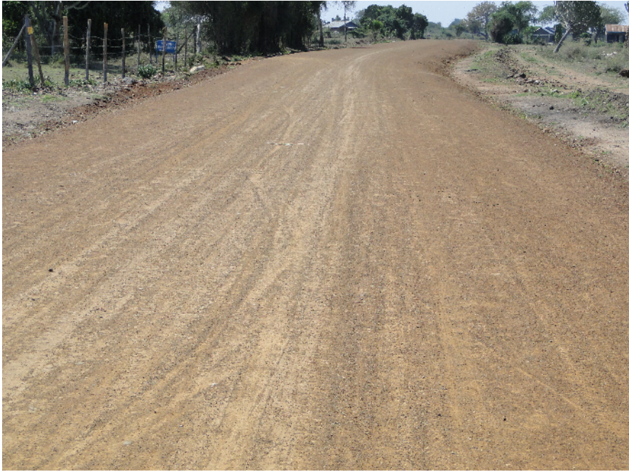
Site clearance and top soil stripping has taken place upto km 14
