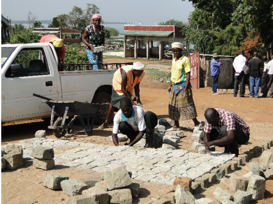
Women participating actively in the laying of a stone base at Uhanya beach
