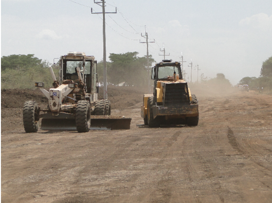
Site clearance and top soil stripping at km16
