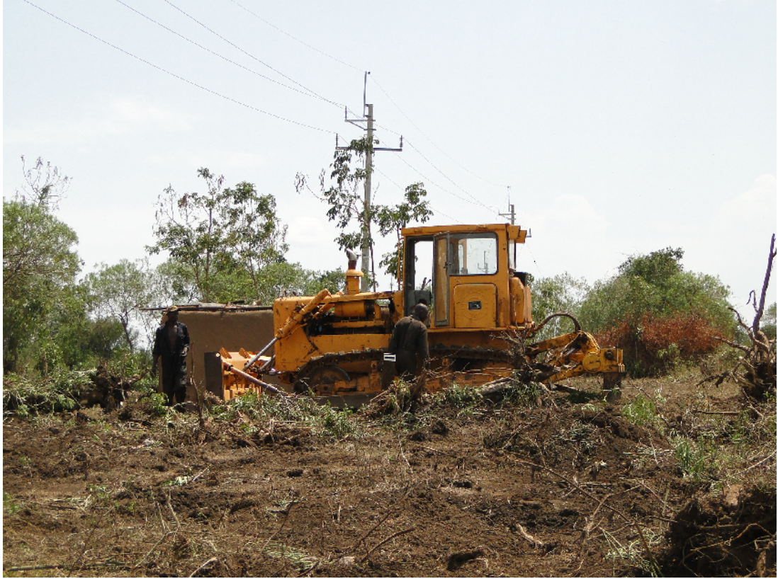
Site clearance at km17
