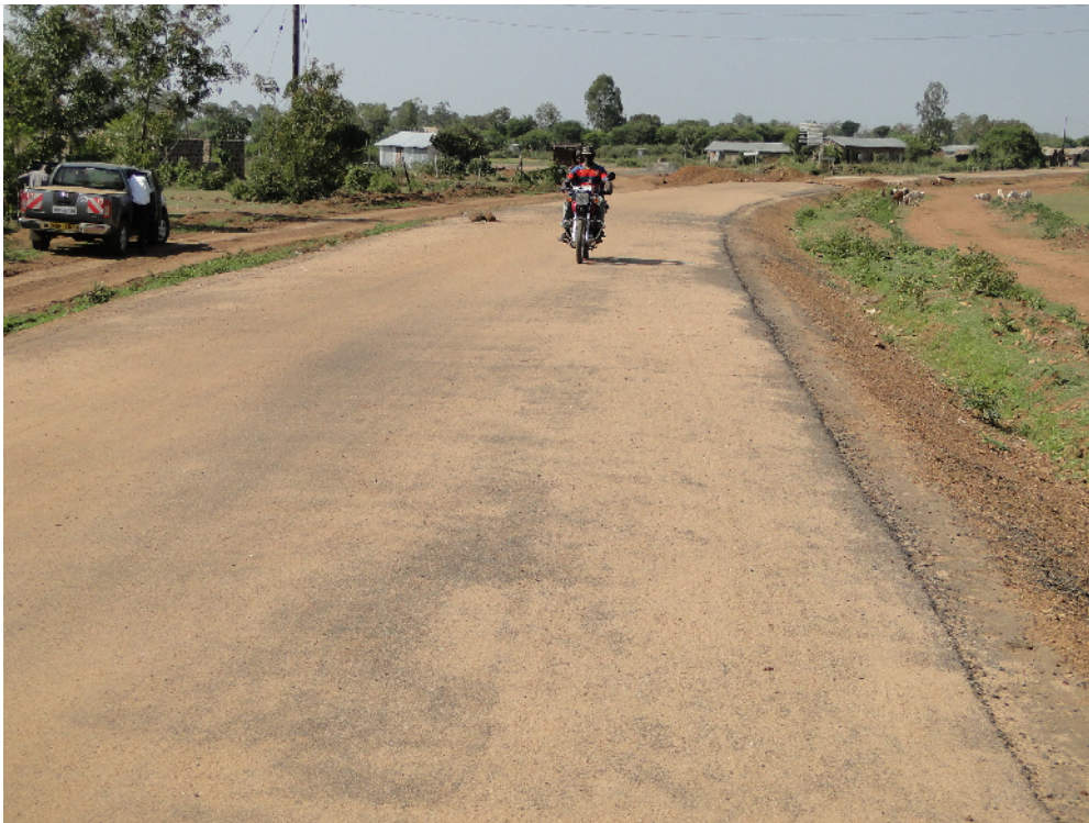
Finished sections of the project between km0-+km1.5
