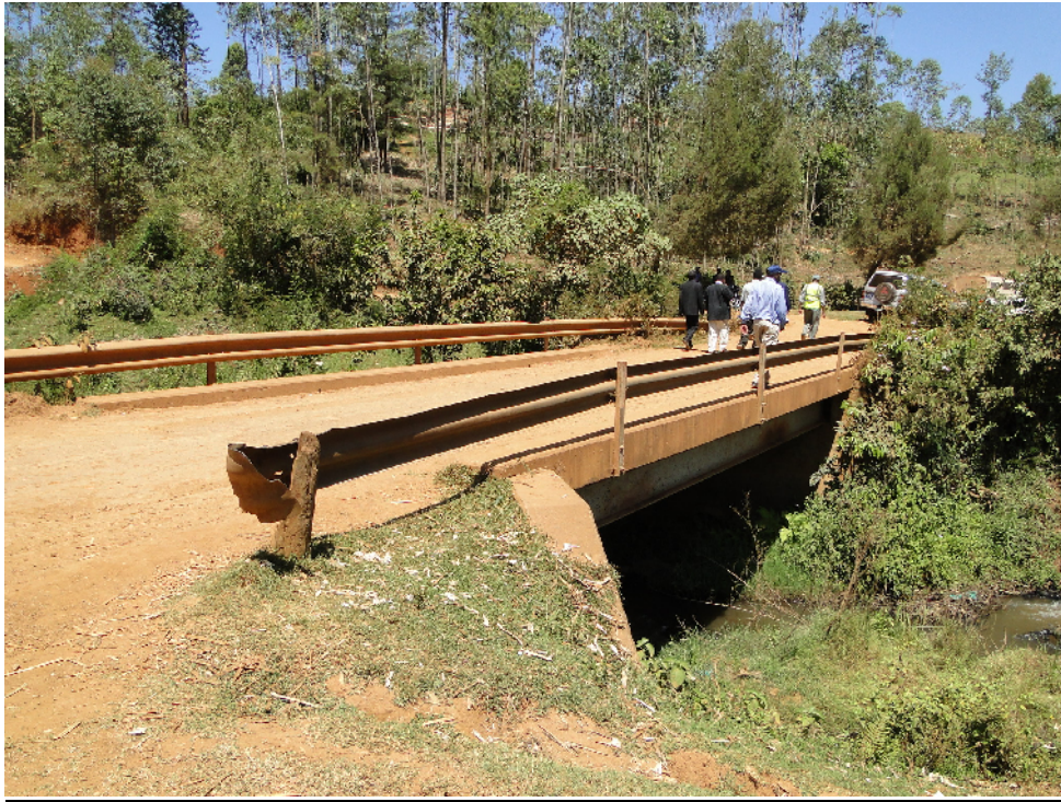
4.4. A bridge earmarked for expansion between km4and km5
