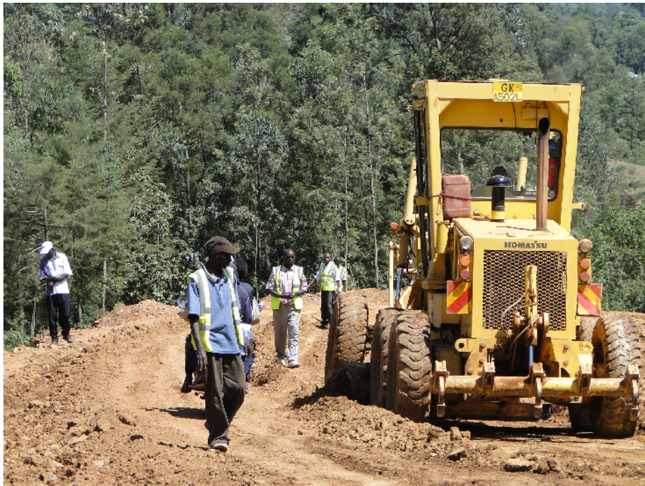
4.3. Grading works taking place at km4
