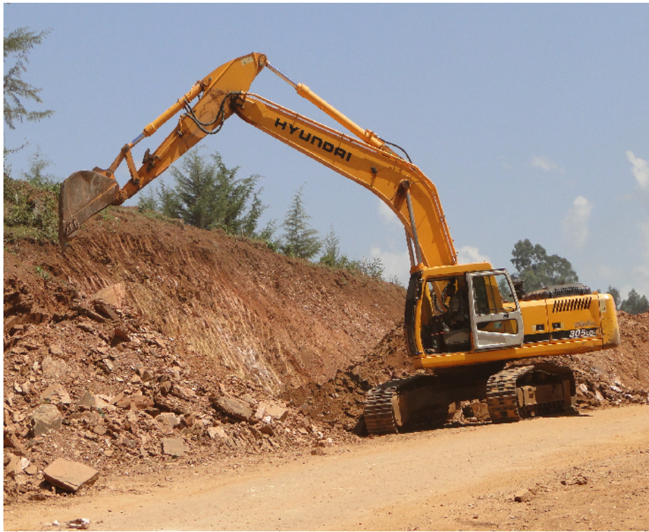
4.5. Excavation to clear the road reserve taking place at km 4.5
