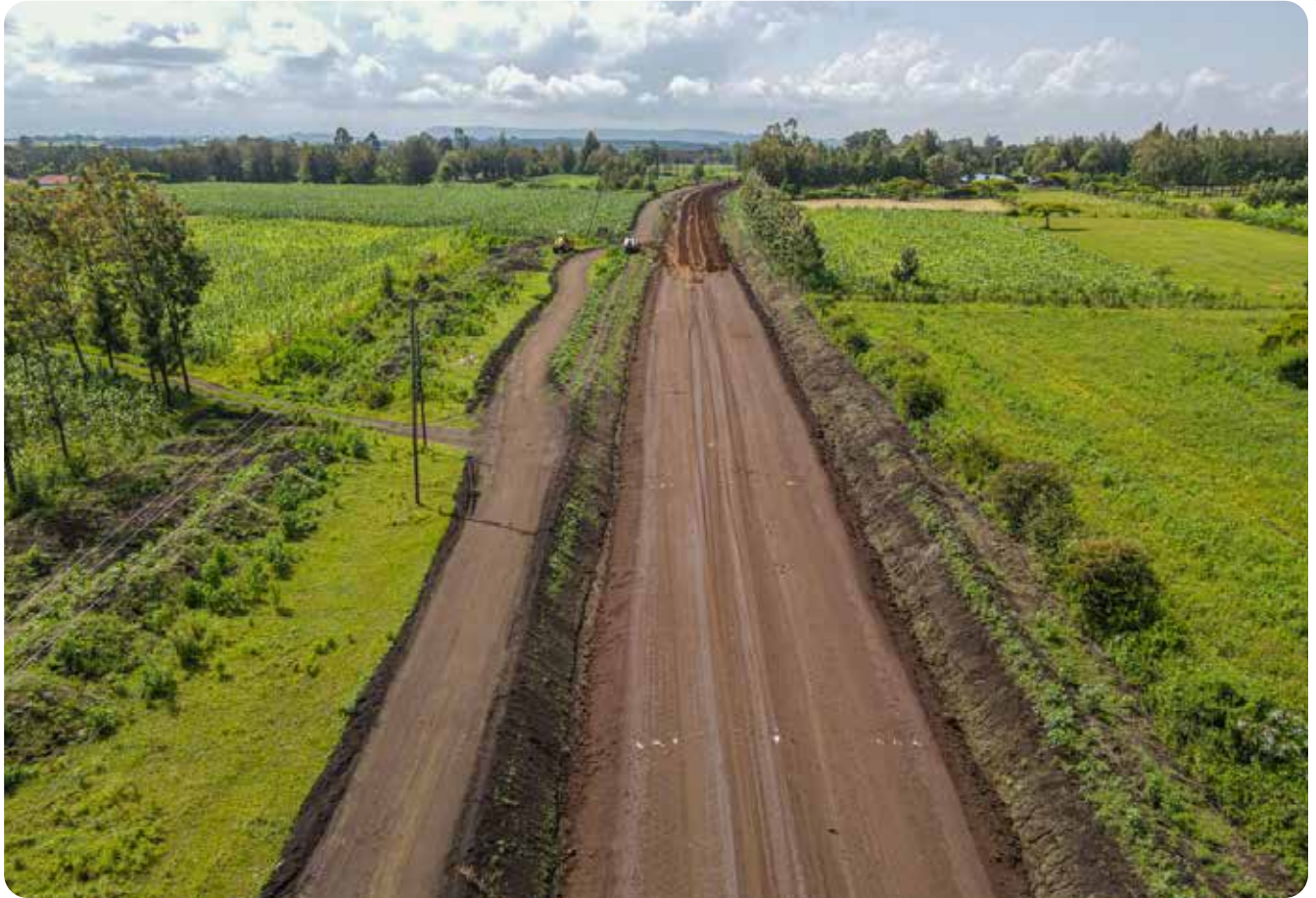
Ongoing Construction of Mercy Njeri Junction B5 Mangu junction D317
