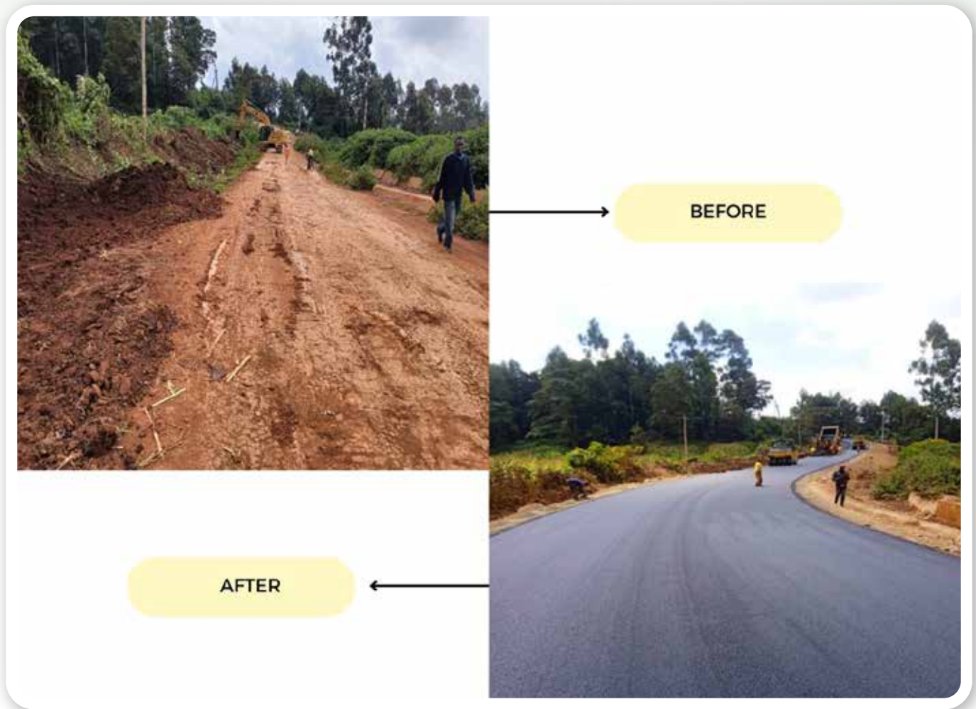
Ongoing Construction of Ngecha-Kanjeru Road project in Kiambu County
