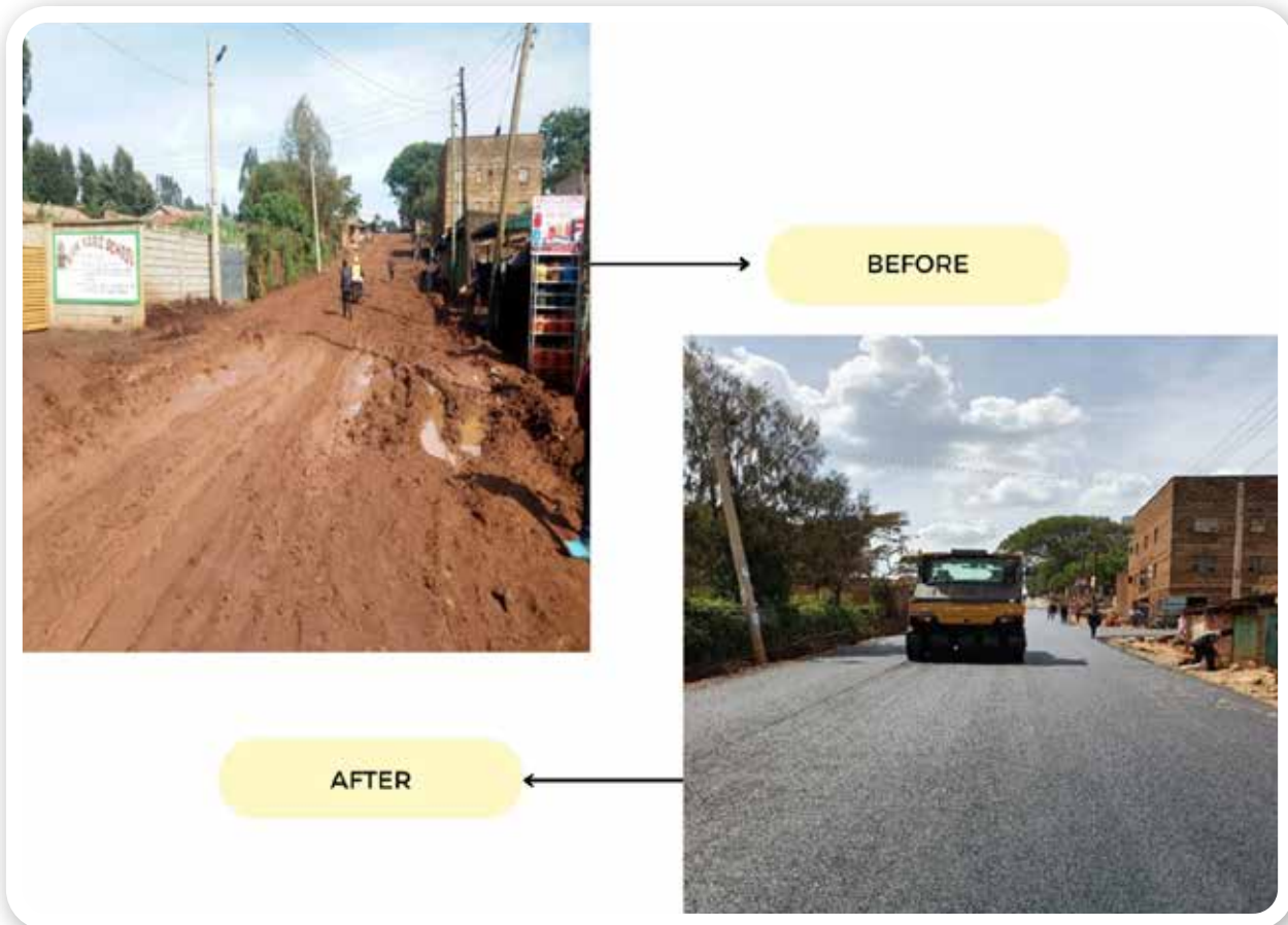
Ongoing Construction of Zambezi-Kiambaa-Gwa Gichini Road project in Kiambu County
