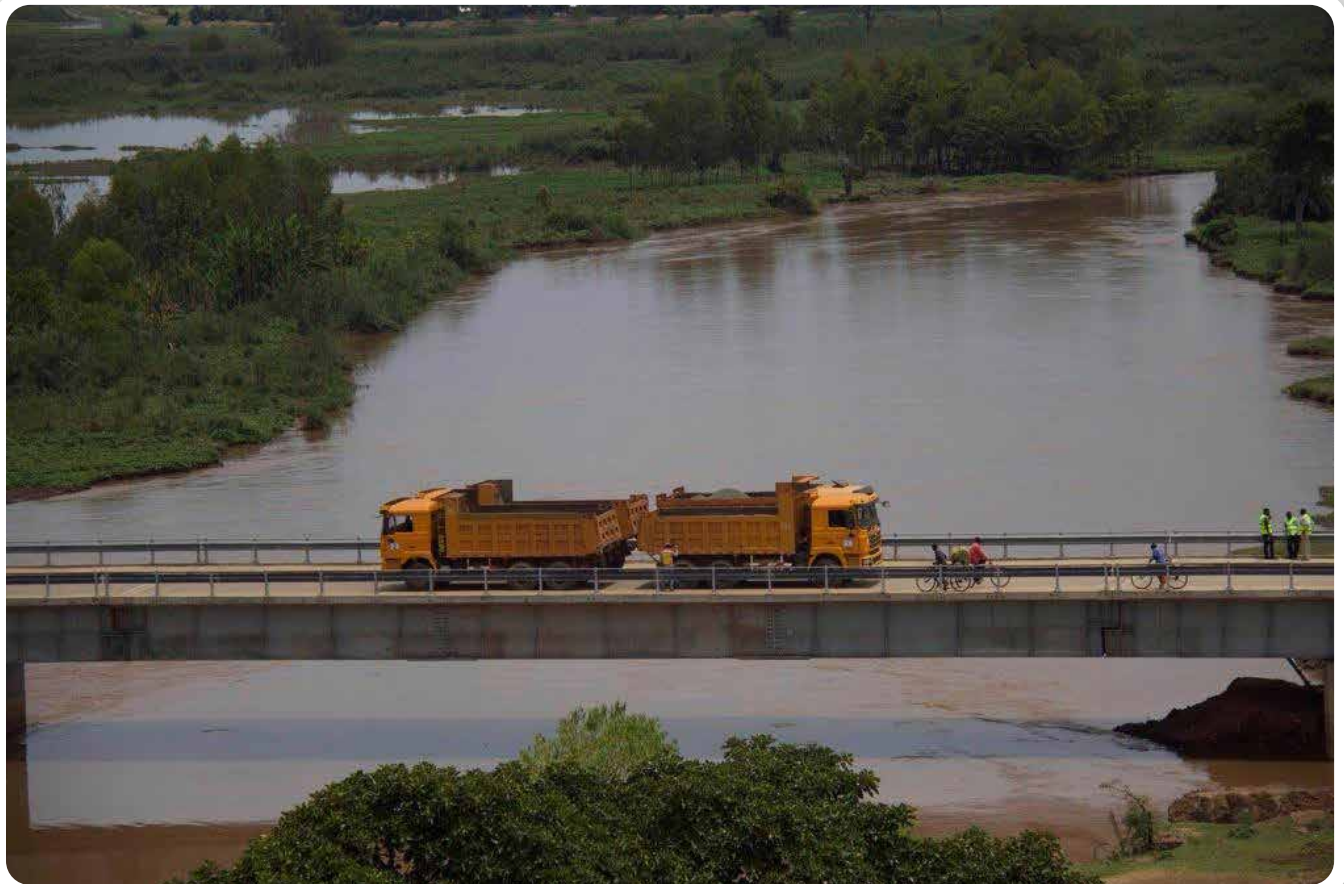
Sigiri Bridge in Busia County facilitating connectivity
